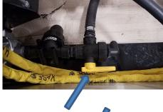
The filter should be cleaned when any noticeable pressure drop is observed.
