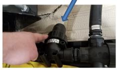
Clean any debris from filter andhousing. Then reinstall.
