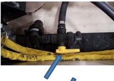
The filter should be cleaned when anynoticeable pressure drop is observed.
