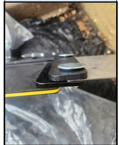
Fig. 4 Block-off plate installation
